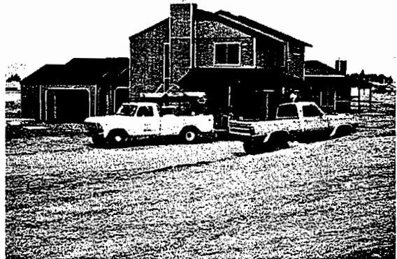
Homes under construction.
